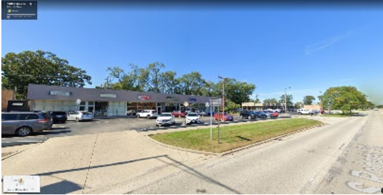
View WB on Roberts Road at Roberts Road and 106 th Street
