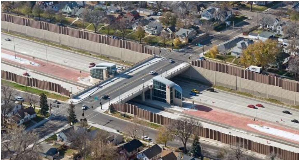
I-35 at 46 th Street, Minneapolis
