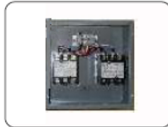
Contactor Panel (088L3441)
