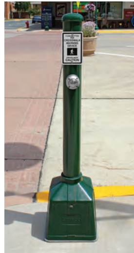
Pedestal pole with push button and base housing wireless communication system
