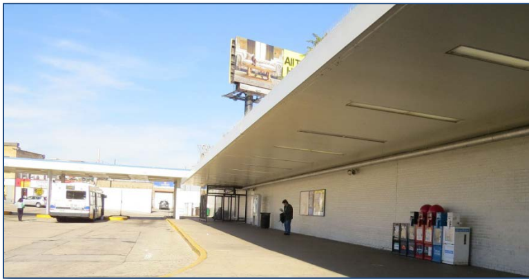
Figure 3.32: CTA Route 68 Bay at Jefferson Park Transit Center
