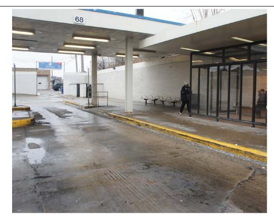
**Photo 2:** Some staining (a de minimis condition) is visible on the pavement in this view of Berth 68, looking north.
