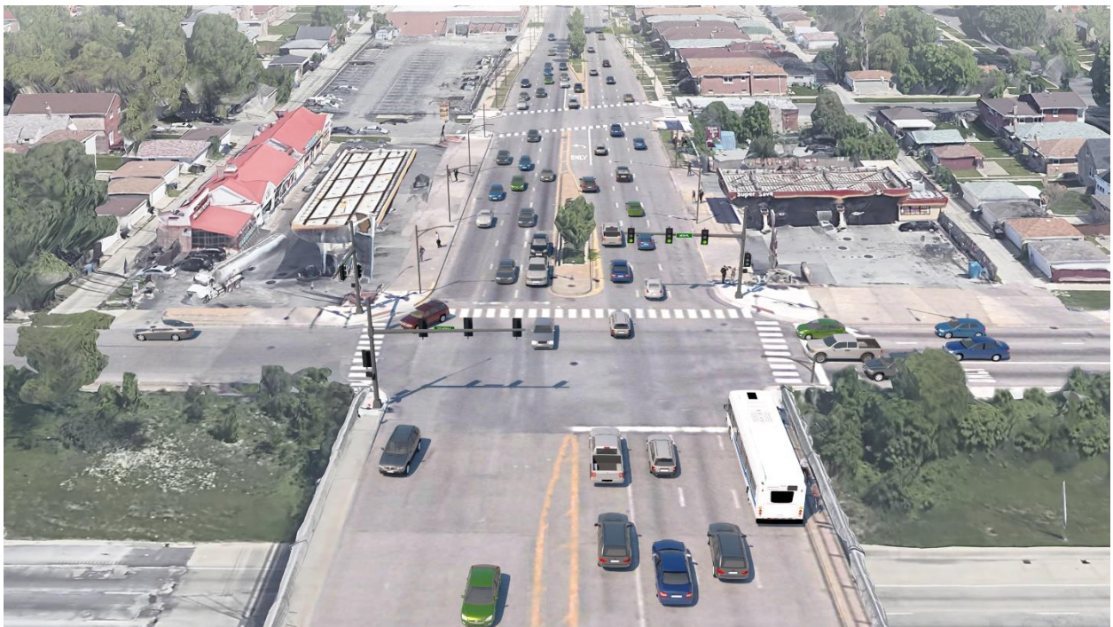
FIGURE 7-5: EXISTING CONDITION OF 98 TH STREET/HALSTED INTERSECTION
