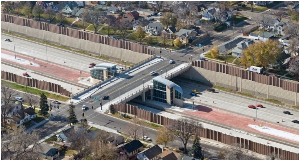
I-35 at 46 th Street, Minneapolis
