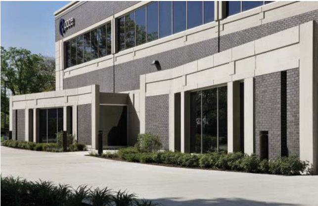
Pace's Administrative Office Building is located in Arlington Heights.
