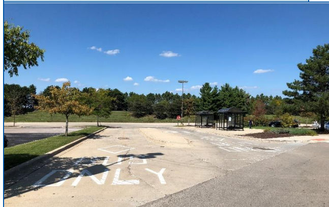
Representative Inspection Photo
