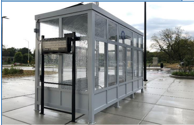
Representative Inspection Photo
