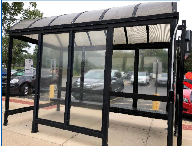
Representative Inspection Photo
