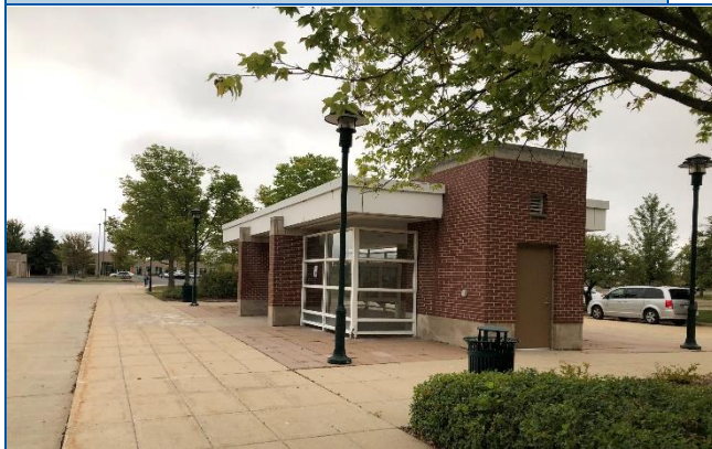
Representative Inspection Photo
